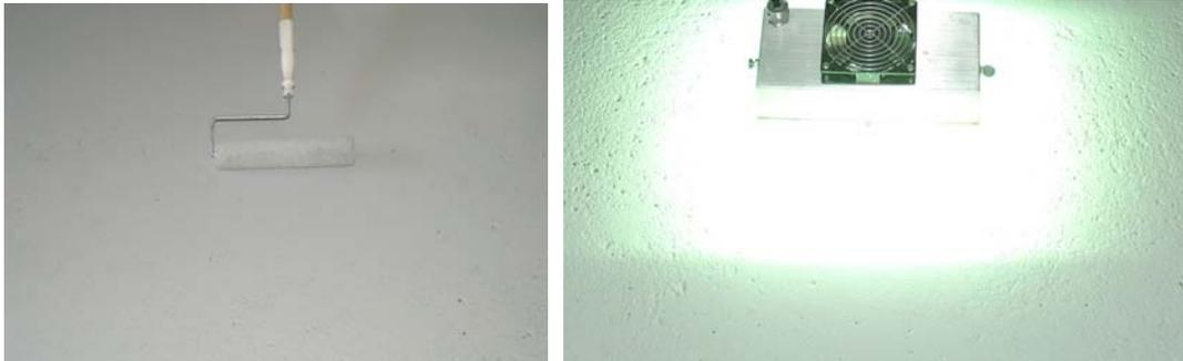
**Figure 2. High Performance UV Technology For Fast Cure Flooring Applications**
