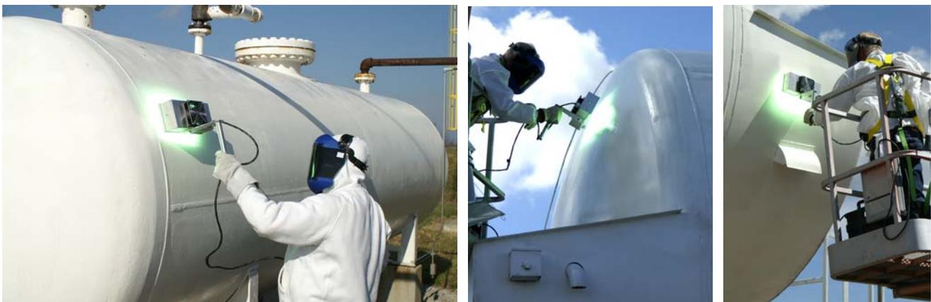
**Figure 3. Field Application And Cure Of High Performance UV Coating Technology**
