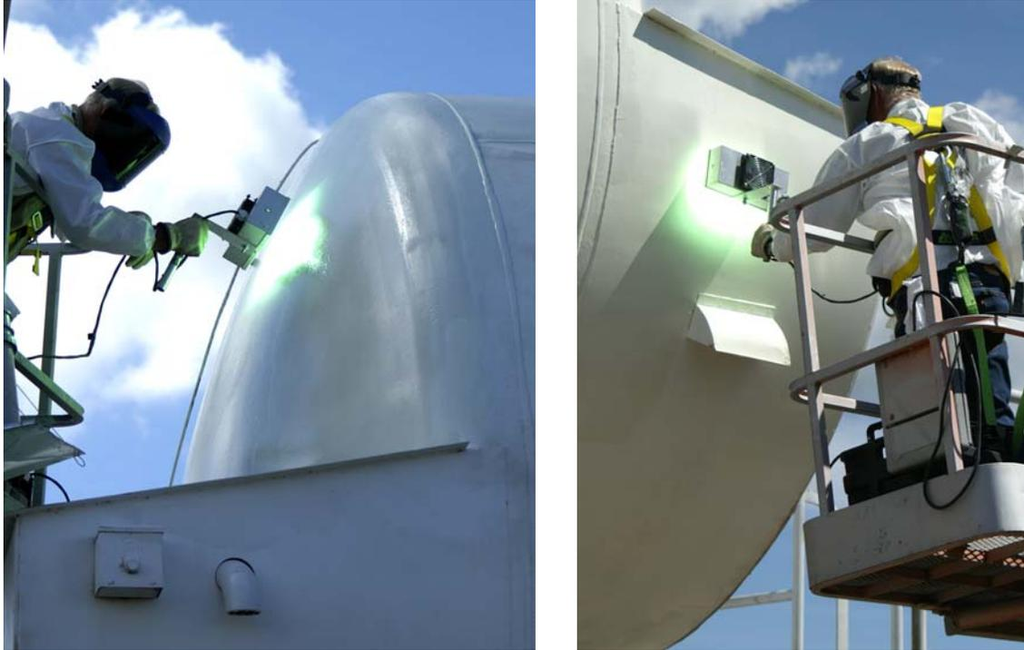
**Figure 2.** Field Application And Cure Of UV Technology At Warm Temperatures
