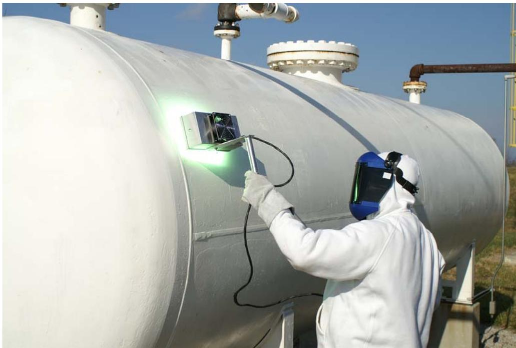
**Figure 1.** Field Application And Cure Of UV Technology At Cold Temperatures
