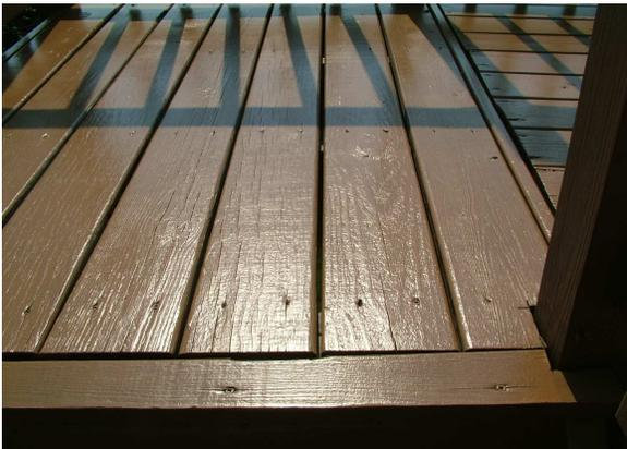
Figure 2: CCA pressure treated southern yellow pine with opaque sealer coat and UV PUD Sunshine PUD
