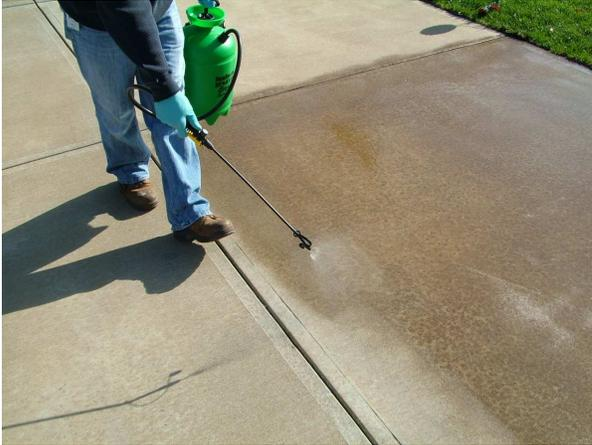
Figure 9 Concrete driveway sealer application
