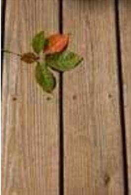
Figure 3: Treated southern yellow pine coated with one coat of a semi-transparent Sunshine PUD
